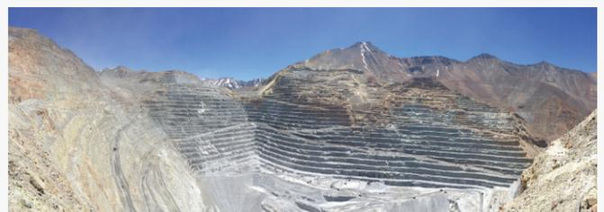
Figure 1: Antofagasta's Los Pelambres open pit is 800m deep and 2km wide.
