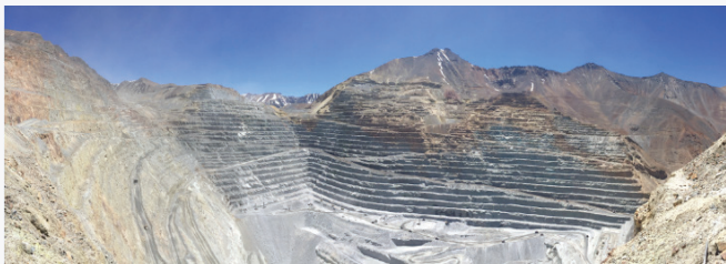
Figure 1: Antofagasta's Los Pelambres open pit is 800m deep and 2km wide.
